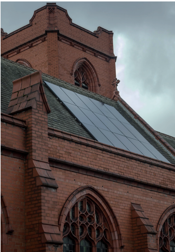
Figure 1: Stage 1 project installed Source: John Hughes
